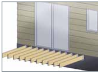
Joists securely attached for better safety
